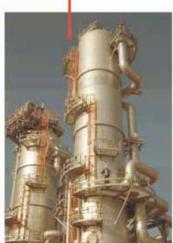
Separation at amine contactor towers
