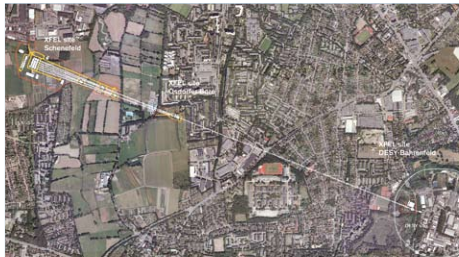
Aerial view of the European X-Ray Laser Facility
